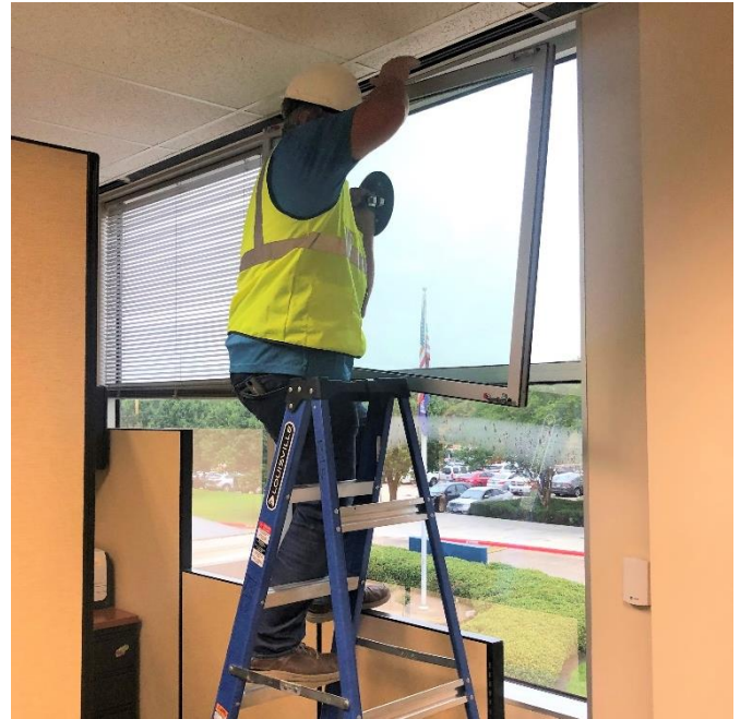
The ultra-lightweight construction of WinSert allows it to be easily installed in minutes without drilled holes or permanent attachment devices.
