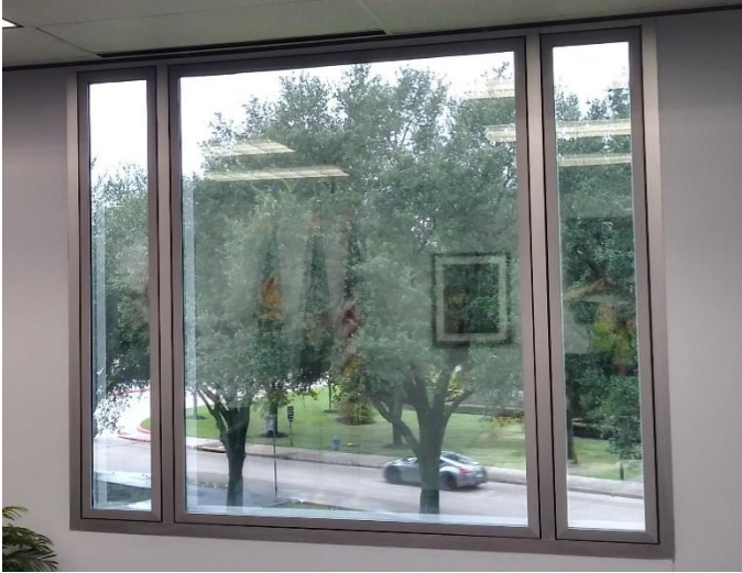
The WinSert Plus secondary window inserts installed into the VA administration building, providing added insulation.
